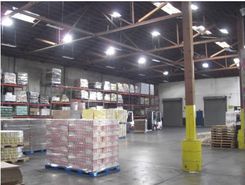
After Light Pipe Installation
